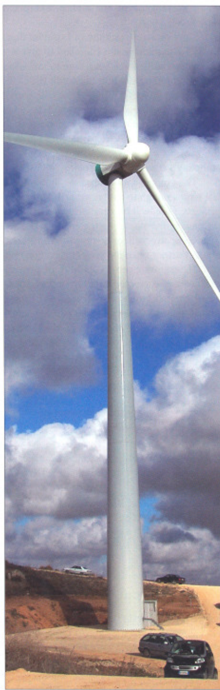
Moncada's prototype: Ready for upgrading from 750 kW to 850 kW
